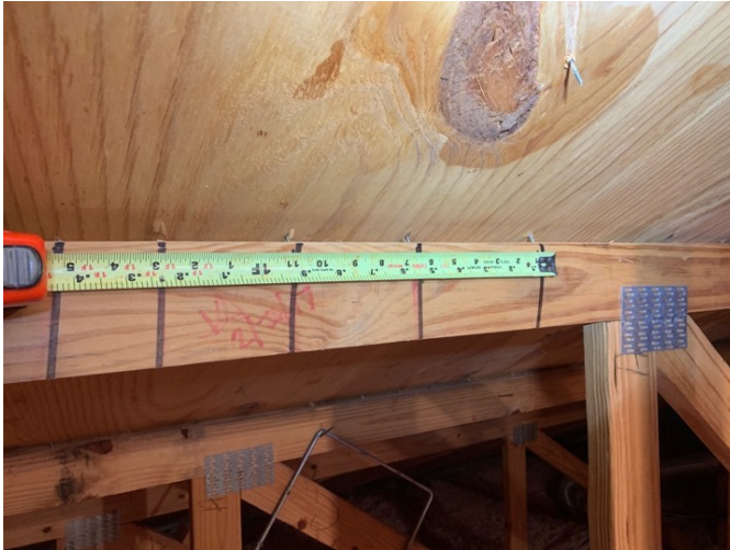
8 penny nails spaced at 6" or less in the field
