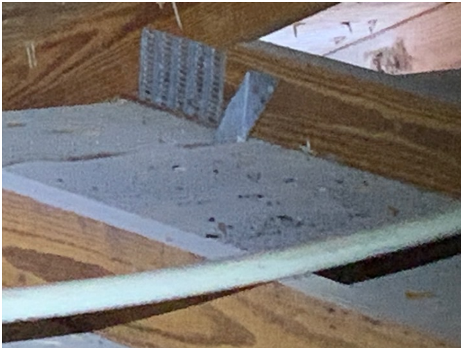
Clips to roof attachments used with 3 nails and attached to topplate
