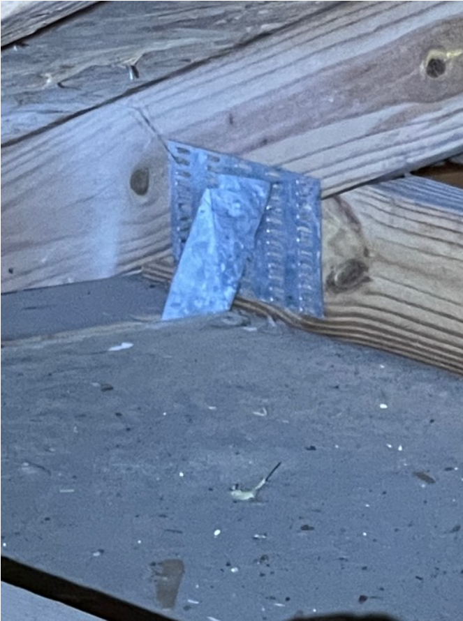
Clips to roof attachments used with 3 nails and attached to topplate
